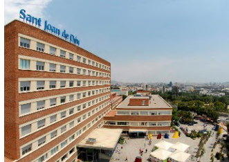
Hospital general pediátrico
